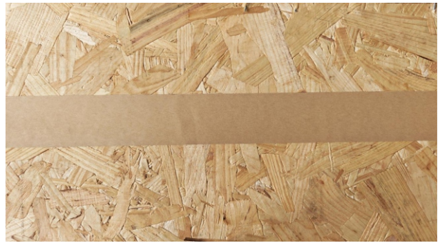
Use VAPOR TAPE adhesive tape to seal flat seams between OSB panels.
