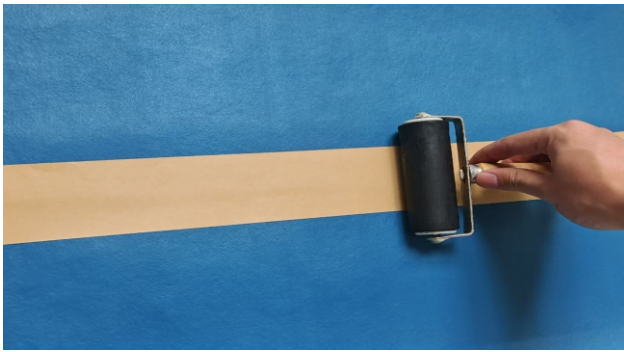
Use VAPOR TAPE to seal overlap ping joints of vapour control layers.
