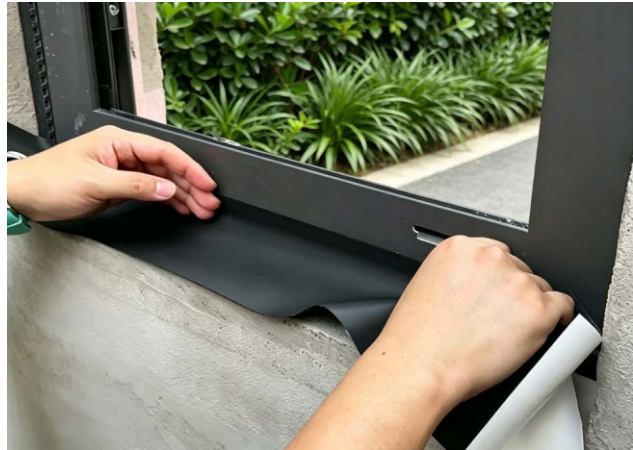
Use EPDM TAPE for perimeter closed-loop sealing of window openings.
