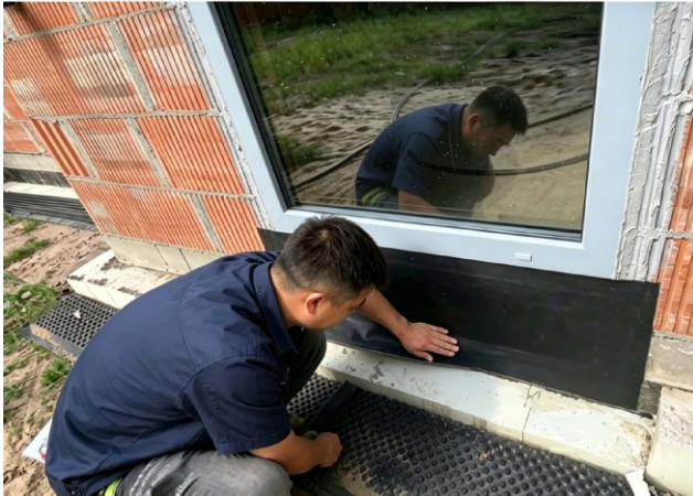
Use EPDM TAPE to perform sealing treatment at the bottom joints of floor to ceiling terrace windows.
