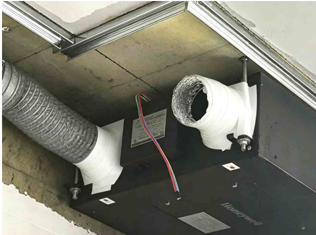
Use WIND TAPE adhesive tape for sealing of circular pipes
