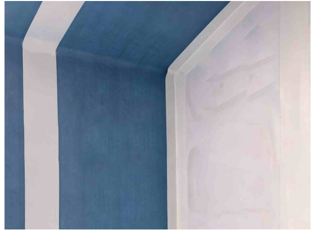
Use WIND TAPE to seal overlap ping joints.
